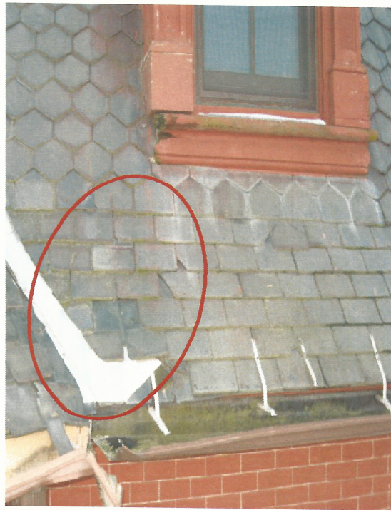
Loose or Missing Slate
