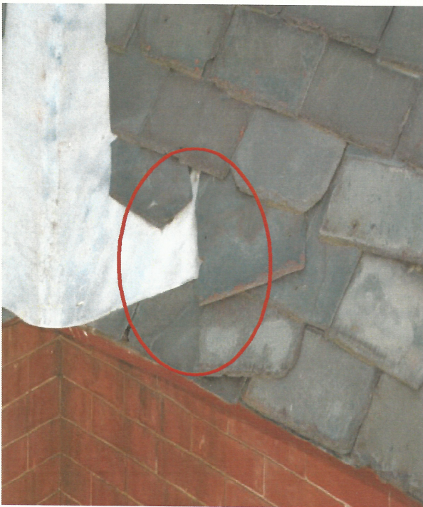
Loose or Missing Slate
