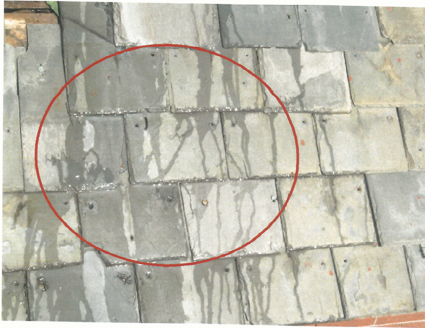
Repairs with used Slates
