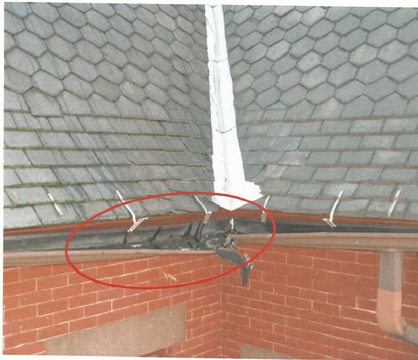
Damaged Gutters
