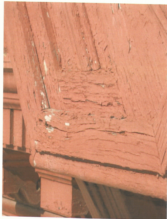
Dried Wood and Peeling Paint
