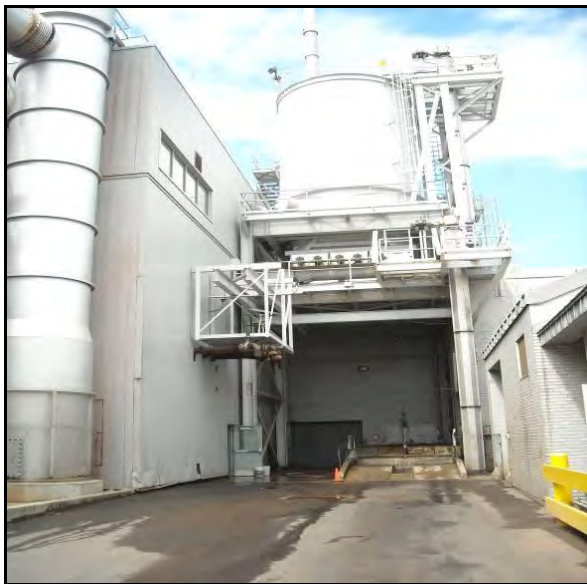
FIGURE 2-20 CAKE STORAGE SILO LOCATED ON THE UPPER LEVEL OF THE FILTER BUILDING AND ENCLOSED SCREW CONVEYORS IN HOT OIL ROOM
