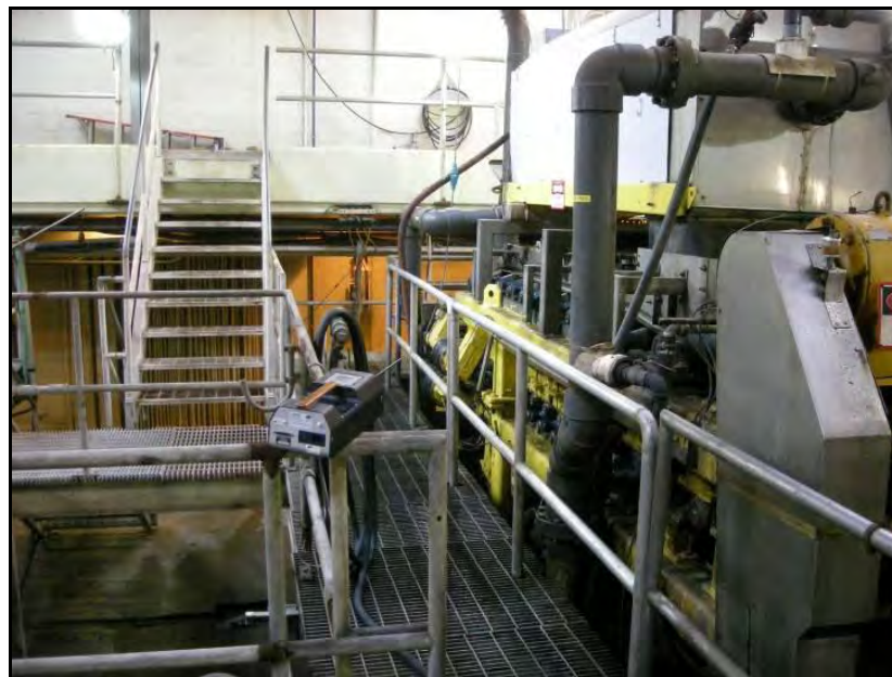
FIGURE 2-17 HYDROGEN SULFIDE MEASUREMENT IN DEWATERING AREA
