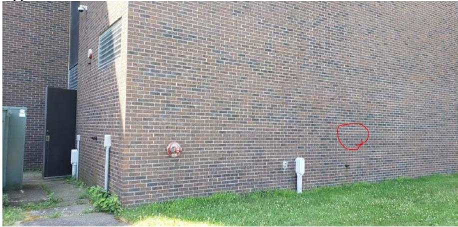
Approximate Location of Meter & Disconnect
