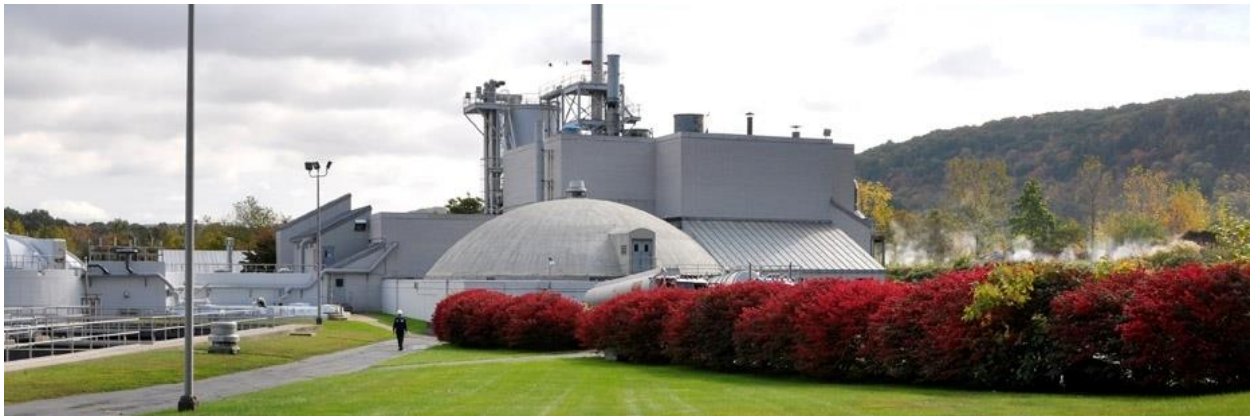
(Photo courtesy of Veolia web site)
