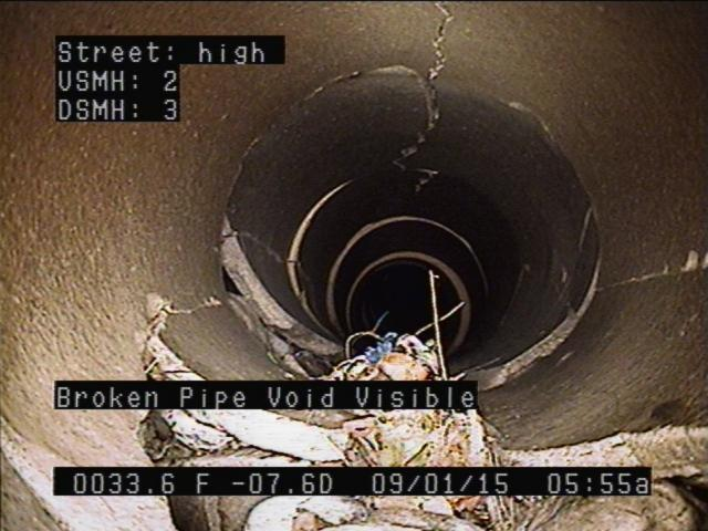
Operator: John City: naugatuck Street: high USMH: 2 DSMH: 3 Direction: Downstream Shape: Circular Material: Vitrified Clay Pipe Height: 15 Width: 15 Access Point Manhole 0000.0 F -07.6D 09/01/15 05:53a
