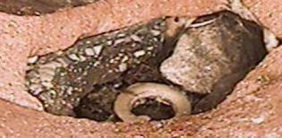
Broken Pipe Void Visible
