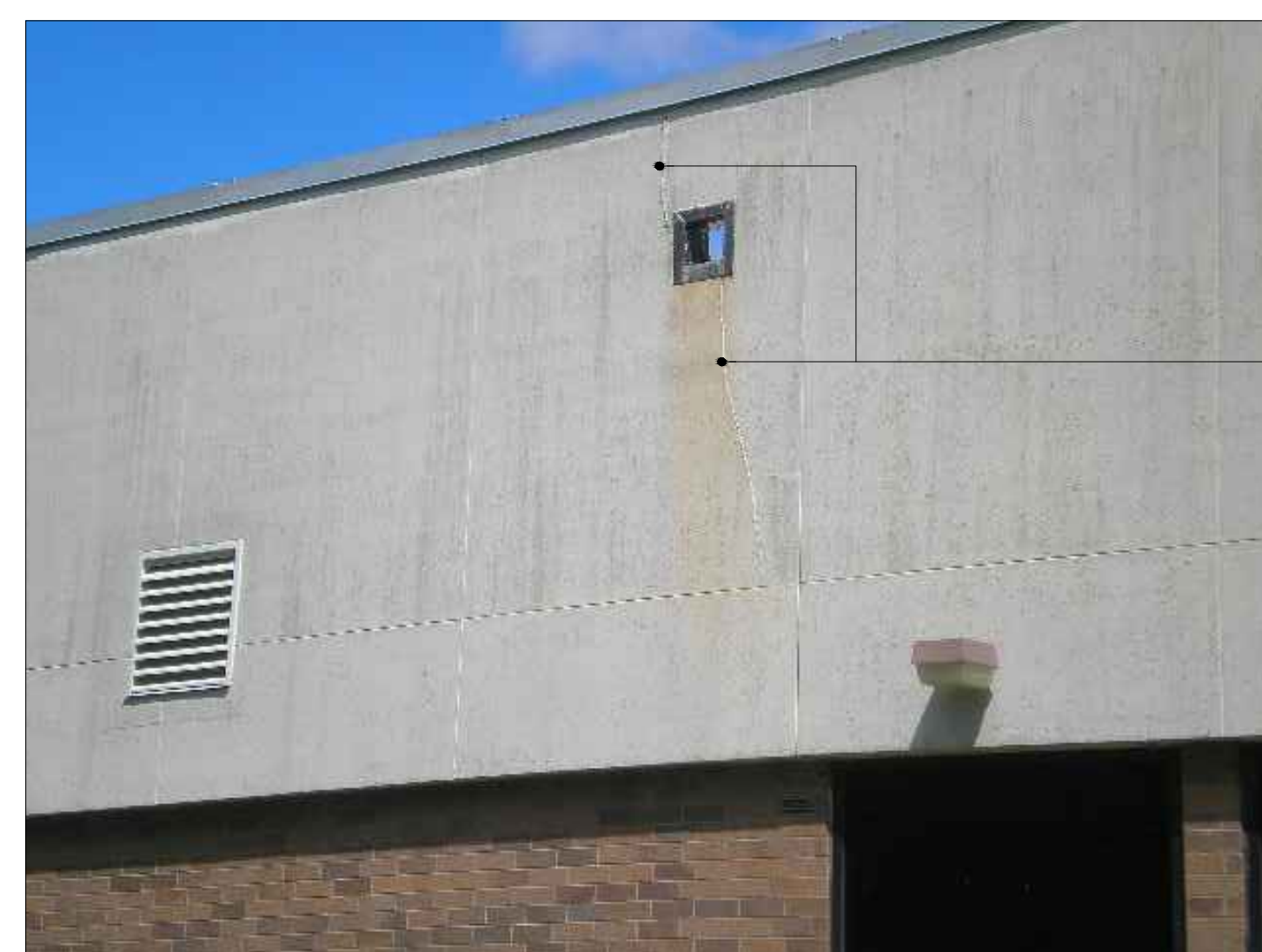
PICTURE #2 @ CRACK IN EIFS SCALE: NONE
